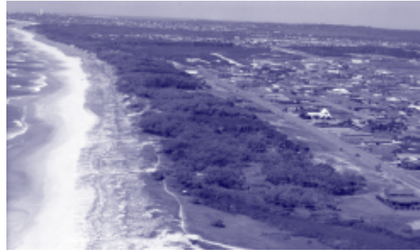
Development has been set well back from the beach at Bokarina on the Sunshine Coast to ensure that the amenity of the beach is always maintained, and so that the development is not threatened by future shoreline movements.
