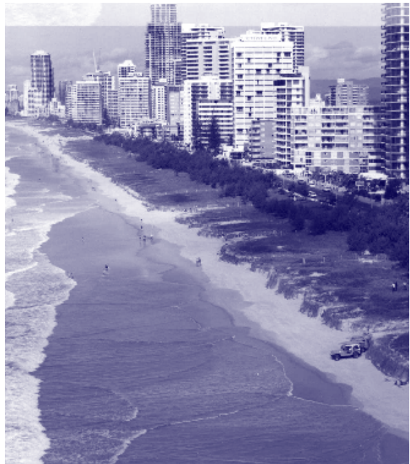
Surfers Paradise beach was nourished with about 1.4 million cubic metres of sand in 1974, and new dunes were formed and vegetated. These dunes have accommodated erosion which occurred during a storm in 1983. The photograph taken soon after the storm shows the beach still in good condition.
